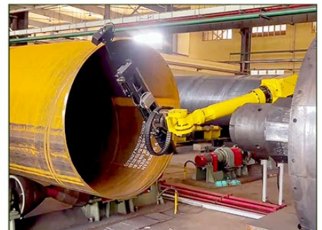
Robot Pipe End Measurement System installed on robot in pipe production
